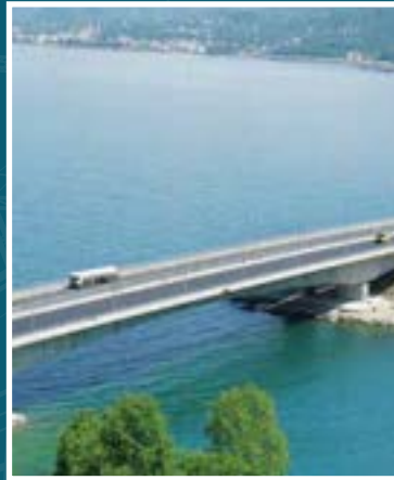
Gölburnu Viaduct, constructed using the Balanced Cantilever Method with Back-Stay, has a total length of 330 meters and is the longest single-span reinforced concrete bridge in Türkiye.
