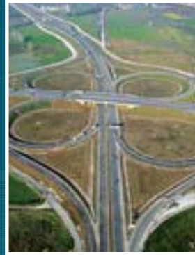
Bursa Ring Road, Yalova Junction- Turanköy Interchange Section, Bursa
