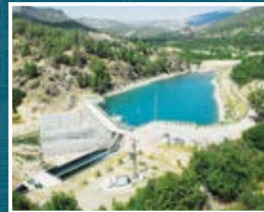
8.89 MW Sarıkavak I Hydroelectric Power Plant Project, Mersin
