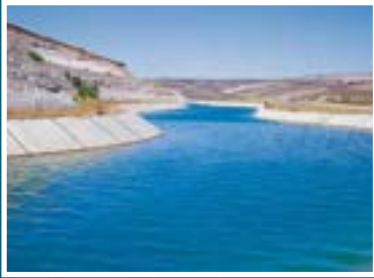
Kralkızı Dicle Gravity Irrigation Transmission Canal Construction, Diyarbakır
