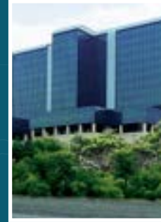
İnönü University Research and Training Hospital Construction, Malatya
