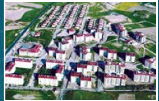
Construction of 462 Housing Units, Ankara
