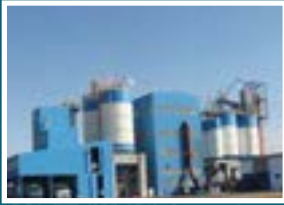
Cement Grinding and Packaging Plant (300,000 Tons/Year), Al-Raqqa/Syria
