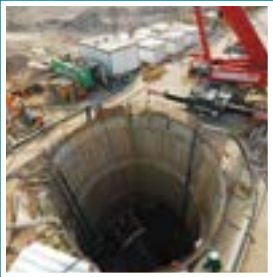
South Jeddah Wastewater Project, Jeddah/Saudi Arabia
